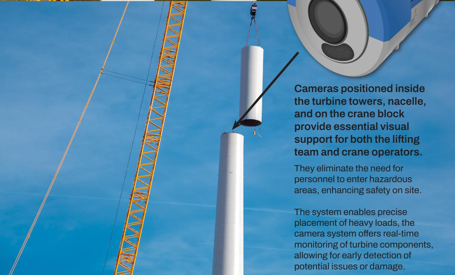
**Cameras positioned inside the turbine towers, nacelle, and on the crane block provide essential visual support for both the lifting team and crane operators.**
